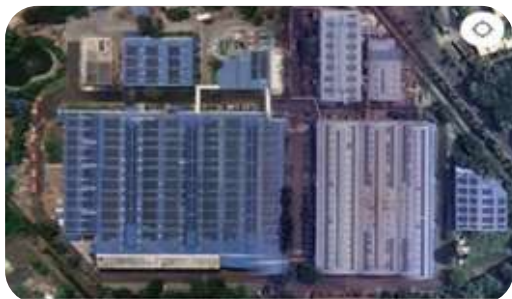
1.02 MW at Mahindra world city unit
