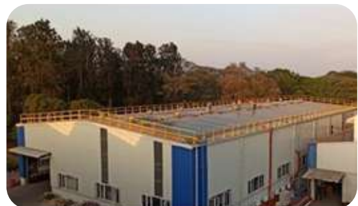
1.14 MW at Hosur unit
